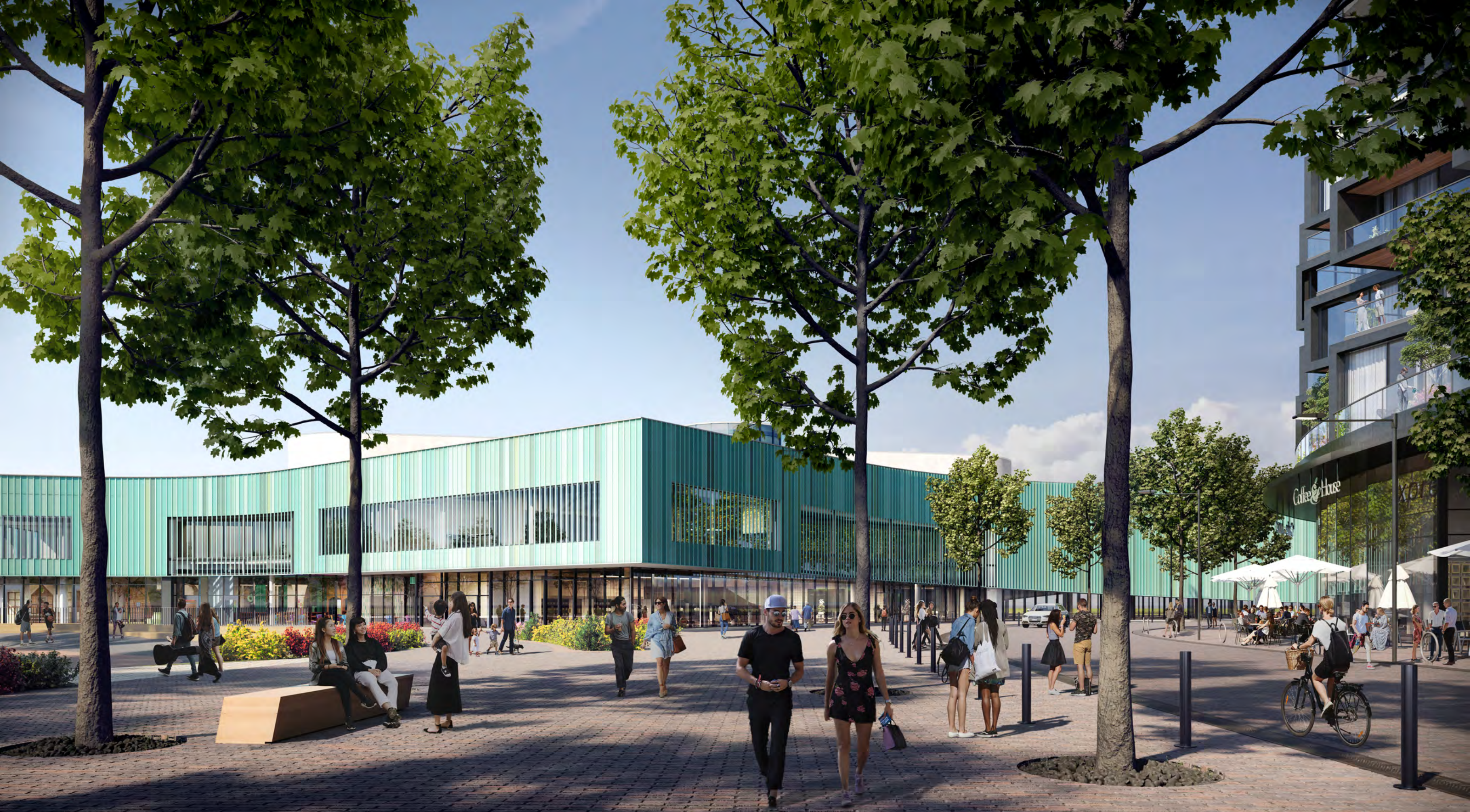
Community Centre planned for Galleria on the Park. Rendering is artist's interpretation only.
